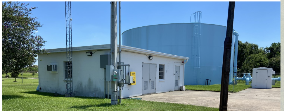
Figure 8-4. Village Drive Water Plant
