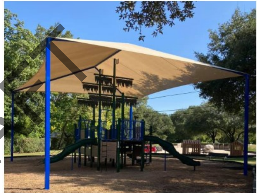
Figure 6-3. Calvin III Ship and shade structure at Carol Fox Park
